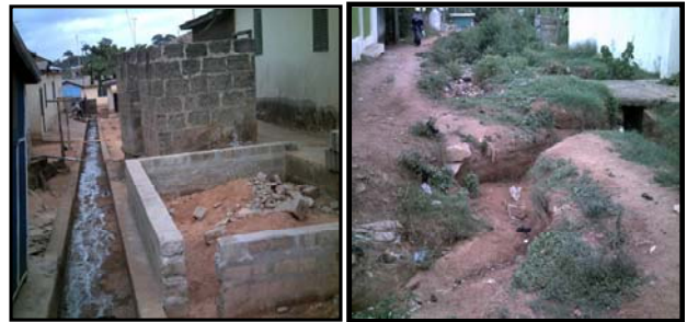
Fig. 6 Encroached and Poor of Roads.
