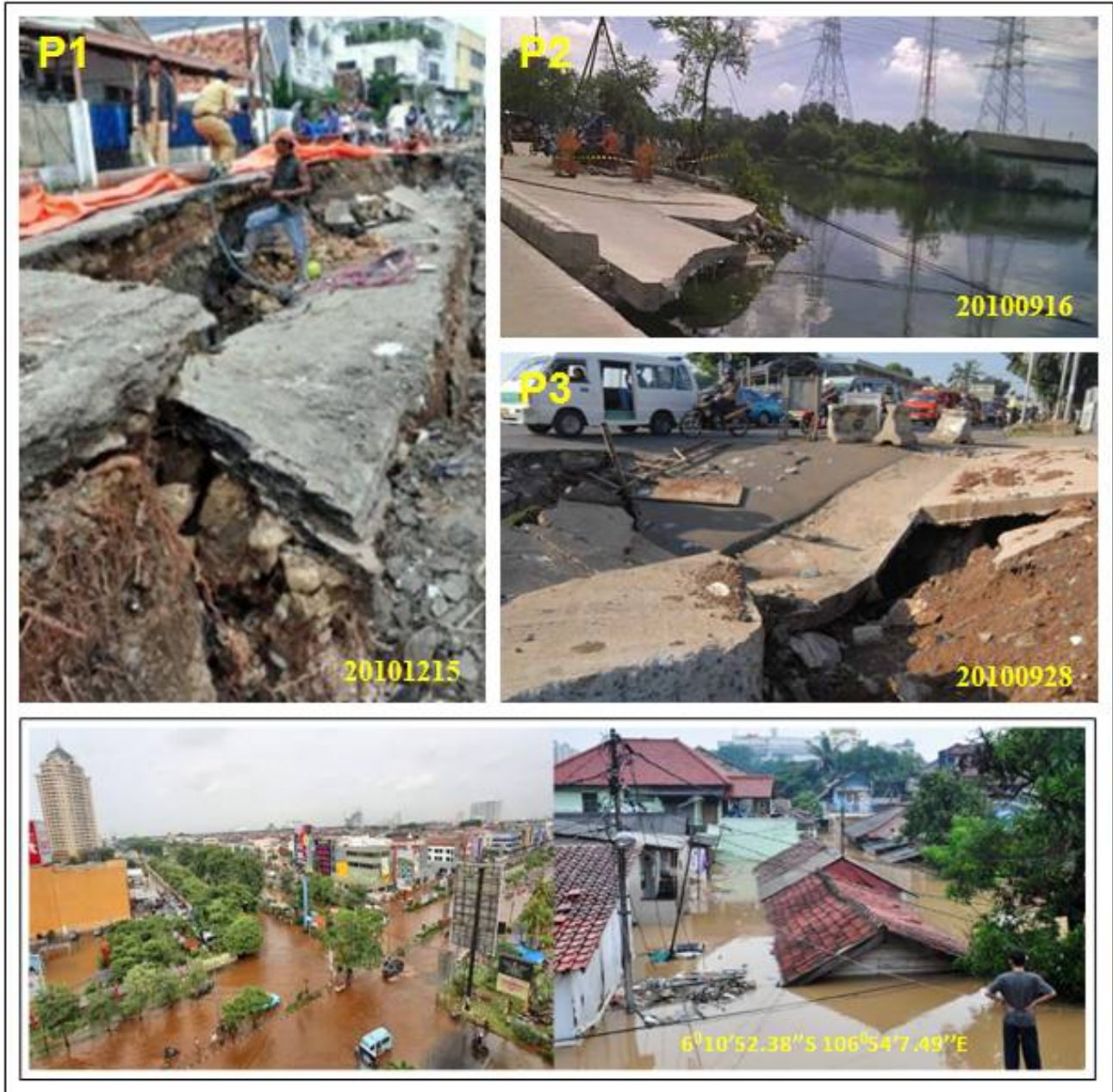
Fig. 9 Land deformation impact areas in northern part of Jakarta urban city: (a) Pantai Utara, (b) Cengkareng, (c) Cakung, (d) Flooding inundation area in northern part of Jakarta urban area in January 2013 as one of land deformation impact and (e) Flooding area in Cakung (P3).
