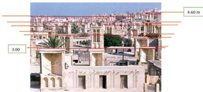
Fig. 10 Higher altitude of wind catcher in central part and their lower altitude on outskirts of Qeshm island
