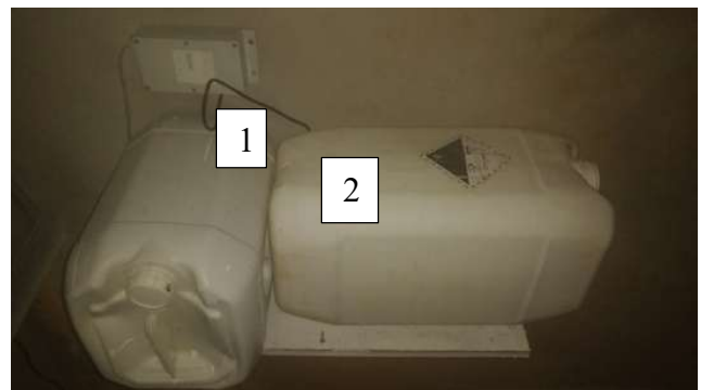
Fig. 3 Grey water reuse reservoirs: (1) 20L; (2) 30L.
