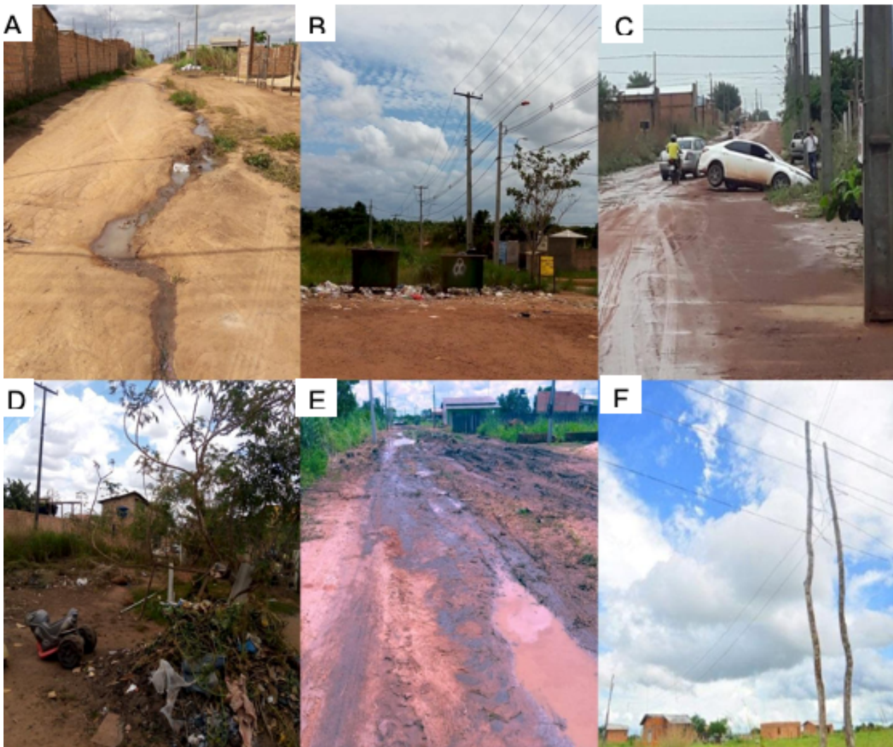
Figure 4. Main problems raised in the interviews and evidenced in the field, such as A) the lack of sanitation, B) poor solid waste collection, in this case, three containers are used for waste disposal in the settlement, C and E) the difficulty of movement due to mud, D) debris in “empty” plots of land and F) clandestine electrical connections.
