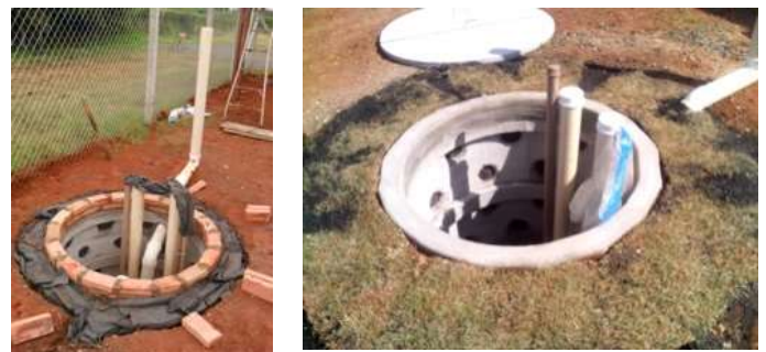
Fig. 4 Experimental dry-well. Source: Ferreira, Reis and Ilha (2016)
