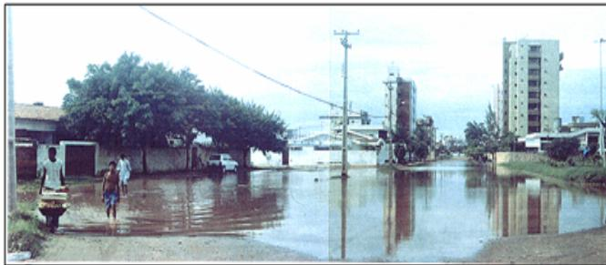
**Fig. 8** Backup damming of natural draining caused by implantation of street networks in 2000. (Nóbrega, 2002)
